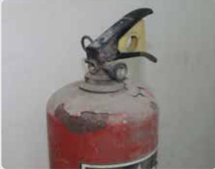
**Colour fading, flaking and rusting** are deterioration signs
