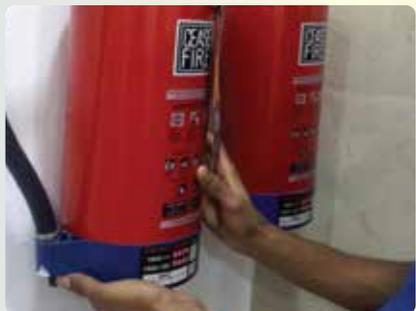
**11.** Installation mounts made of superior grade metal are designed after our extensive research in the field. The unique J Brackets hold the extinguisher firmly in spite of the weight, yet with an easy turn of the angle, enables the extinguisher to detach at the time of need.
