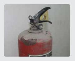
Colour fading, flaking and rusting are deterioration signs
