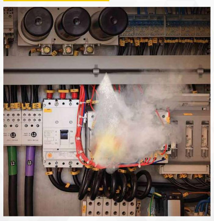
IN-PANEL TUBE BASED MICRO-ENVIRONMENT SUPPRESSION SYSTEM (CQRS)
